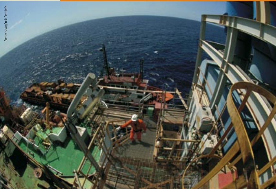
Worker at the platform P-34
